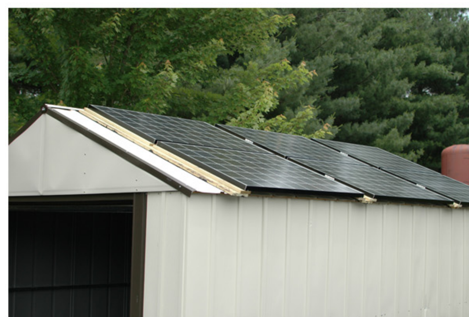
Test Building showing 6 Kyocera KD180GX-LP Panels
