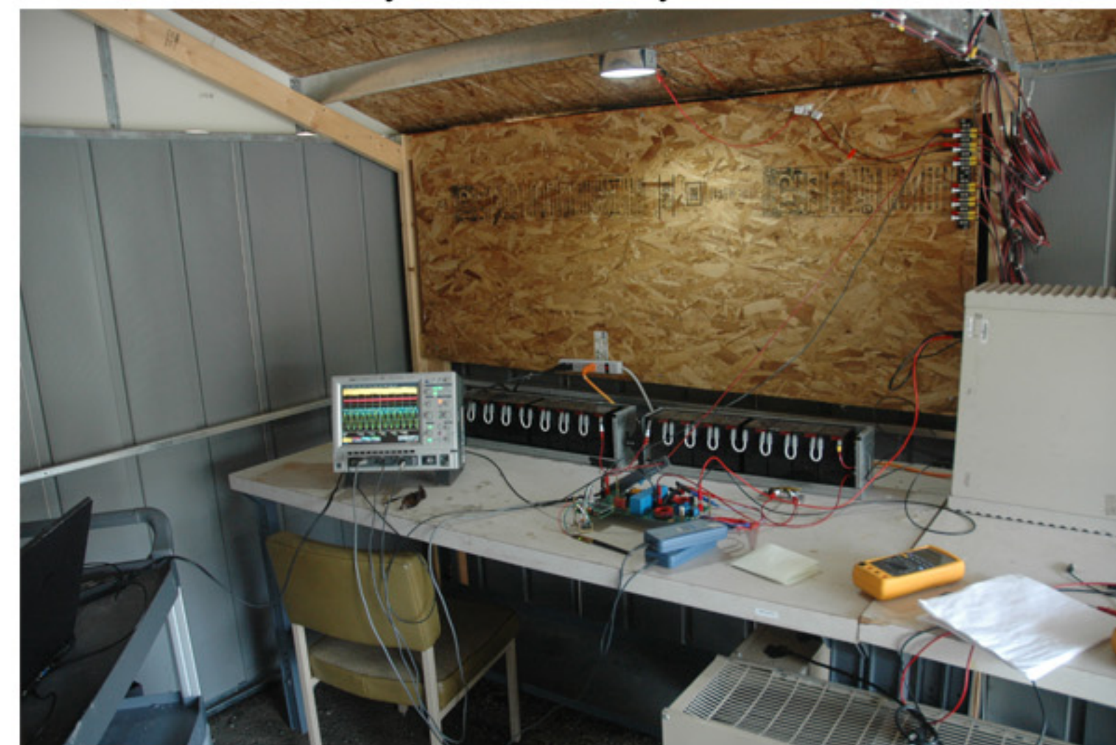
Test Setup showing single-unit with resistive load and battery-stack clamp for DC-bus.
